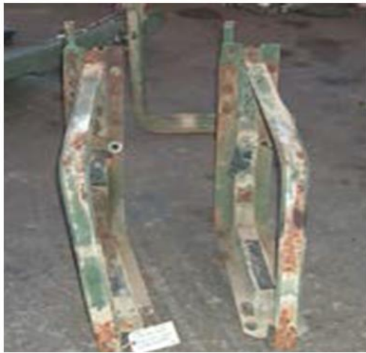
Figure 34: Corrosion of the MTRV Fuel Tank Straps
