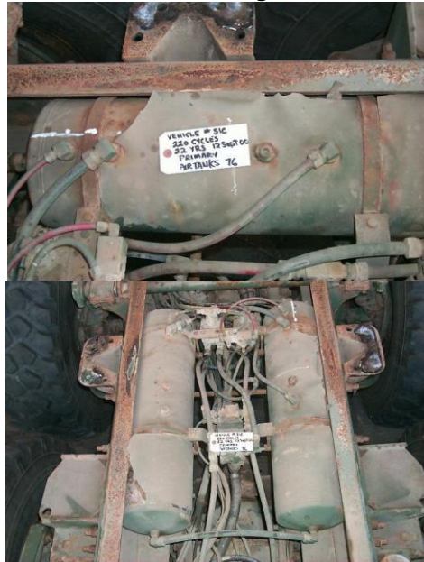
Figure 43: MTRV Air Tanks and Frame Coating Deterioration during ACDRT
